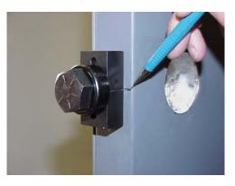
The use of the two steel bars (supplied) and C clamps (not supplied) will help prevent door distortion when forming latch pocket. Clamp one on the inside and outside edge of door as shown.
