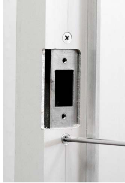
Finished installation showing strike and dust box.
