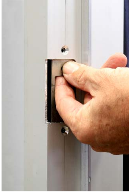
Factory mounting bracket being installed.
